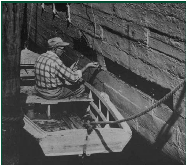
The Captain Is Also the Carpenter. Captain Heath of the Jeanie D. Bell replaces a rotted plank.
