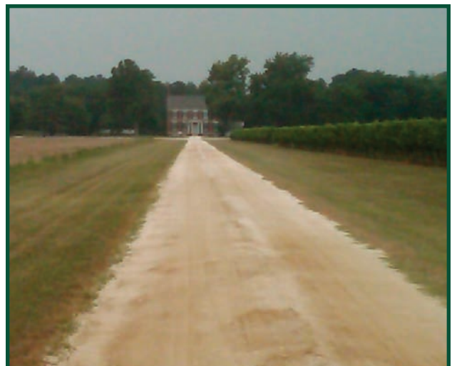
Shell roads like this one were made of crushed oyster shells. Image courtesy of Frank J. Morgan.
